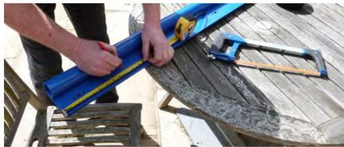
2. To reduce the AquaSpoiler ensure you cut equal amounts from both sides of the centre section only.
